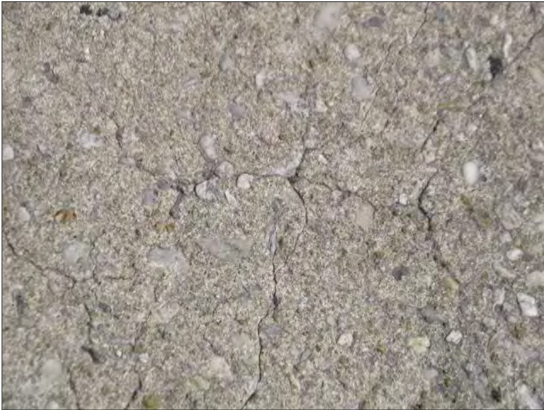
HAIRLINE MAPCRACKING IN DECK IN ALL SPANS
