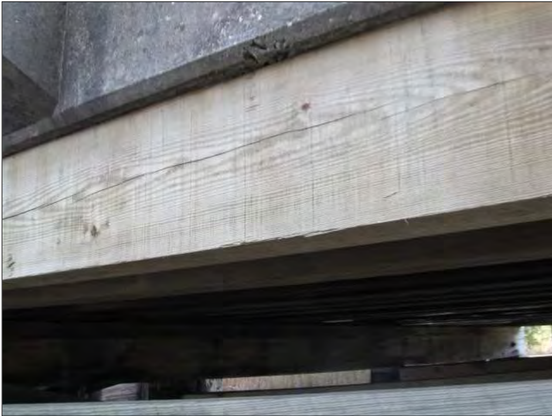
JOIST 1 IN SPAN 1 REPLACED WITH CCA MATERIAL
