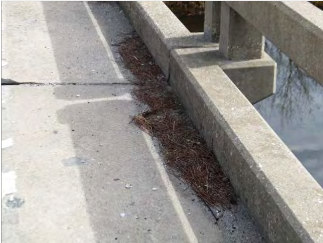
DEBRIS ALONG SOUTH CURB BLOCKING DRAINS
