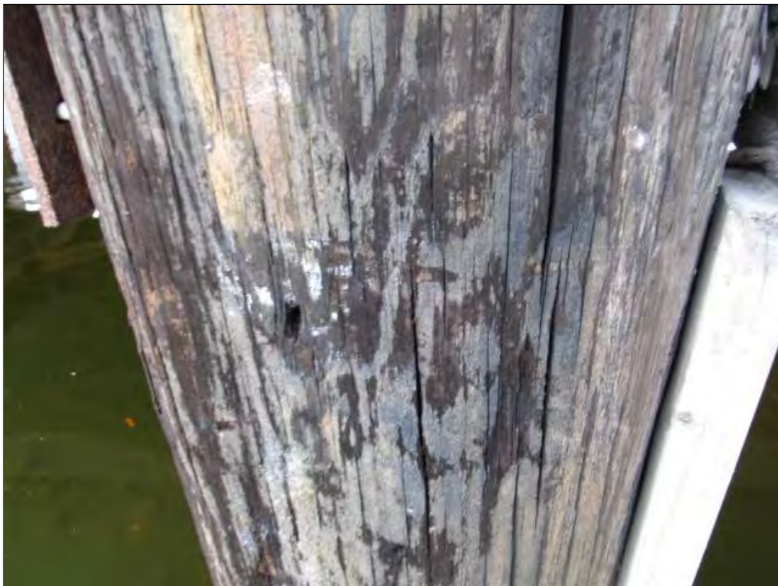
LONGITUDINAL CRACKING ALONG TIMBER PILES UP TO 1/8" WIDE
