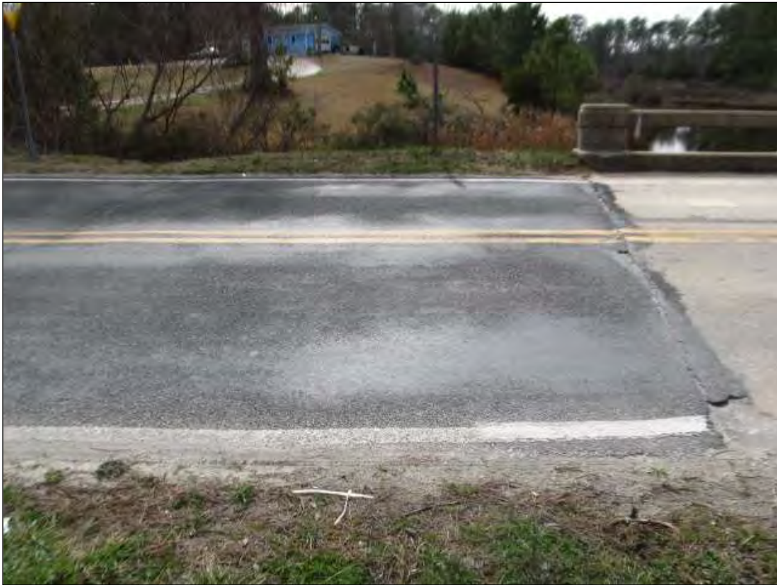
EAST APPROACH ASPHALT WEARING SURFACE SETTLED 1"
