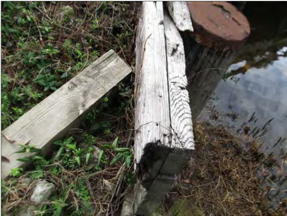
NORTHEAST WINGWALL BOARDS DECAYED AT END PORTION
