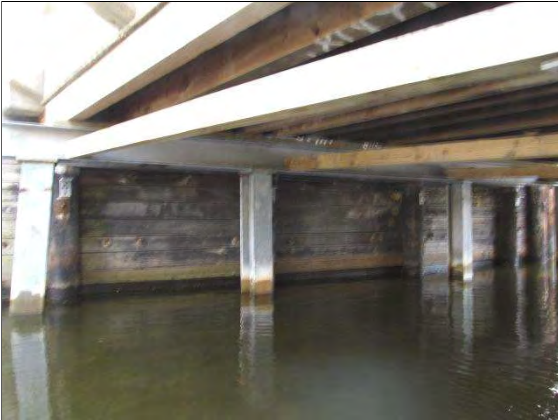
STEEL CRUTCH BENT IN PLACE AT END BENT 2
