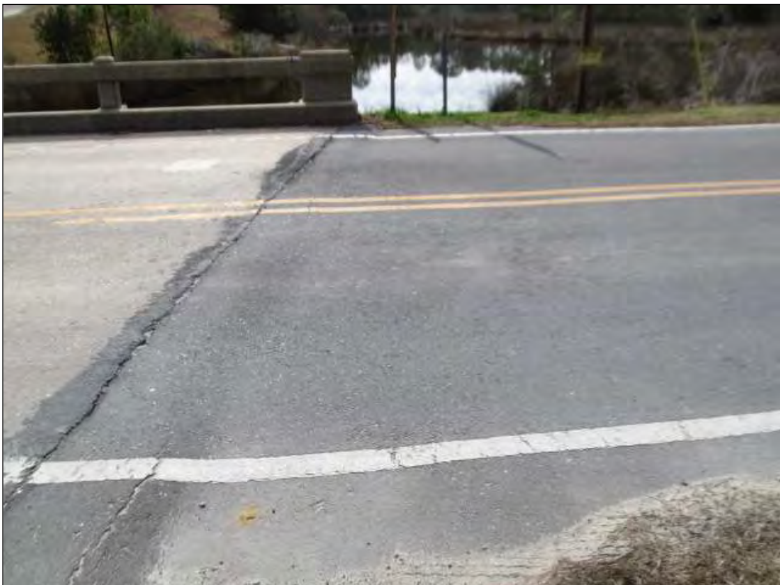
WEST APPROACH ASPHALT WEARING SURFACE SETTLED 2"
