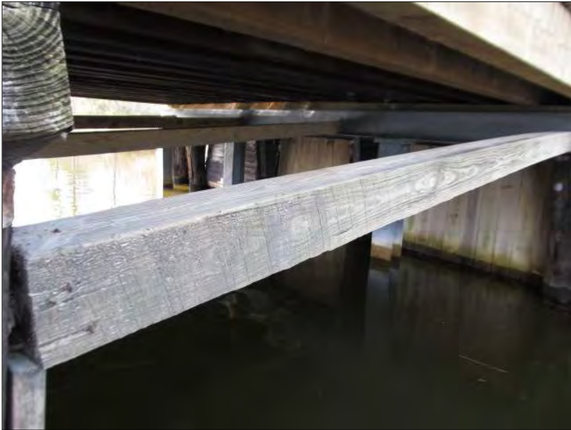
LONGITUDINAL BRACING IN PLACE AT BENT 1 PILES IN SPAN 1 SIMILAR AT BENT 2 IN SPAN 3 AND SPAN 2.
