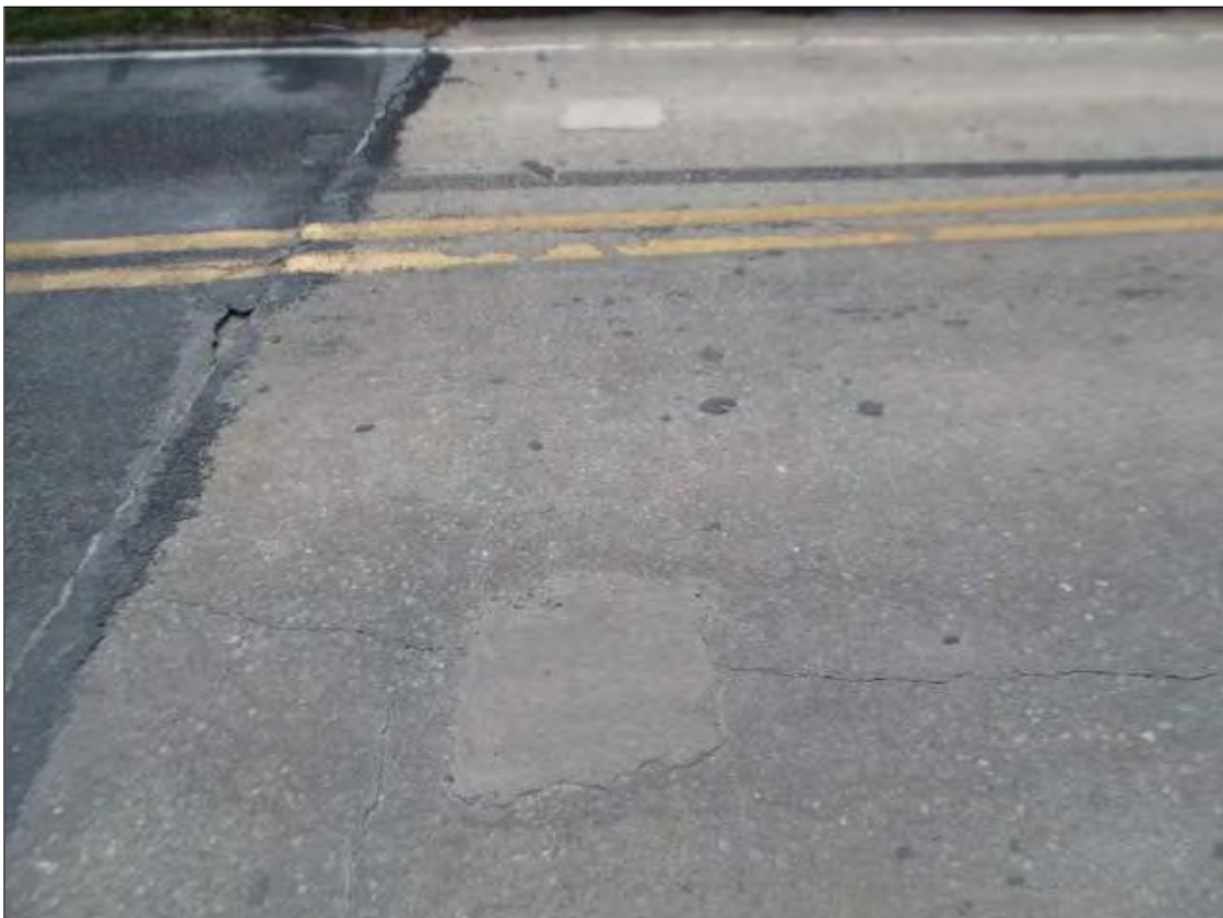
PATCHES IN SPAN 3 DECK AT EAST END
