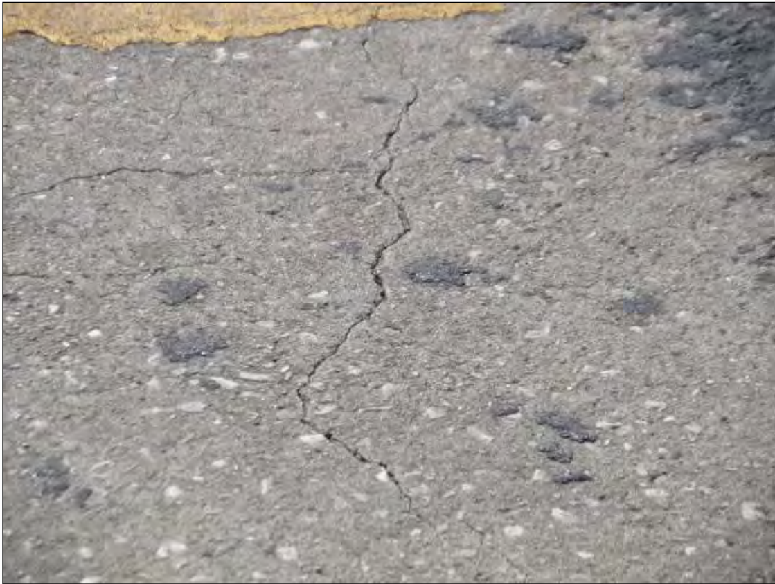
TRANSVERSE CRACKING IN DECK OVER END BENTS UP TO .020" WIDE
