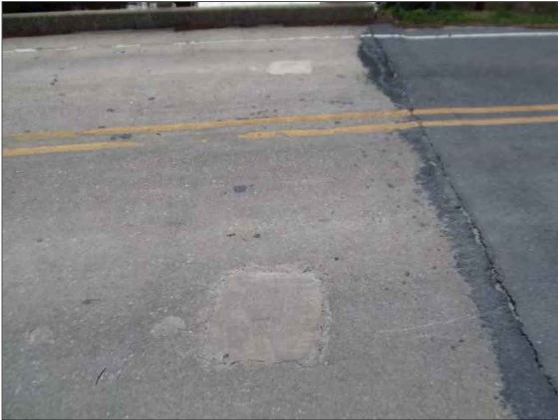
PATCHES IN SPAN 1 DECK AT WEST END
