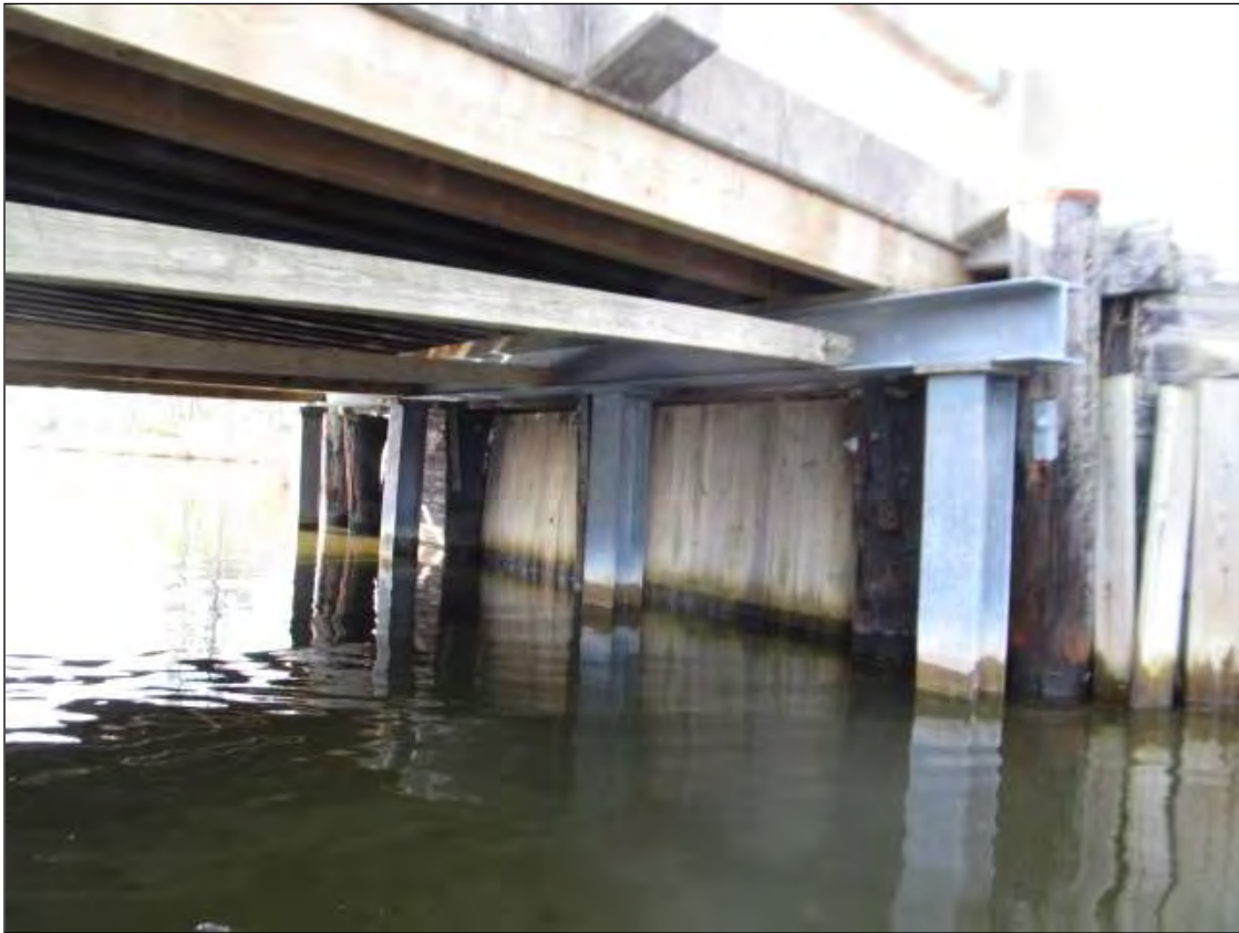
STEEL CRUTCH BENT IN PLACE AT END BENT 1
