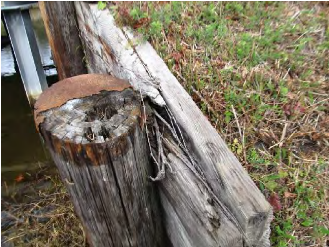
SOUTHEAST WINGWALL BOARDS DECAYED AT END PORTION
