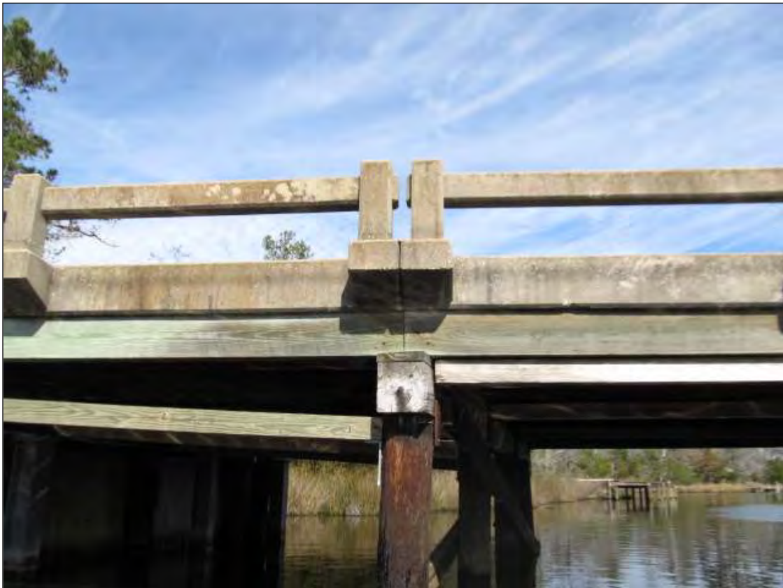
SOUTH END OF BENT 1
