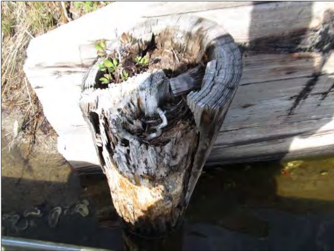
SOUTHWEST WINGPILE DECAYED AND HOLLOW
