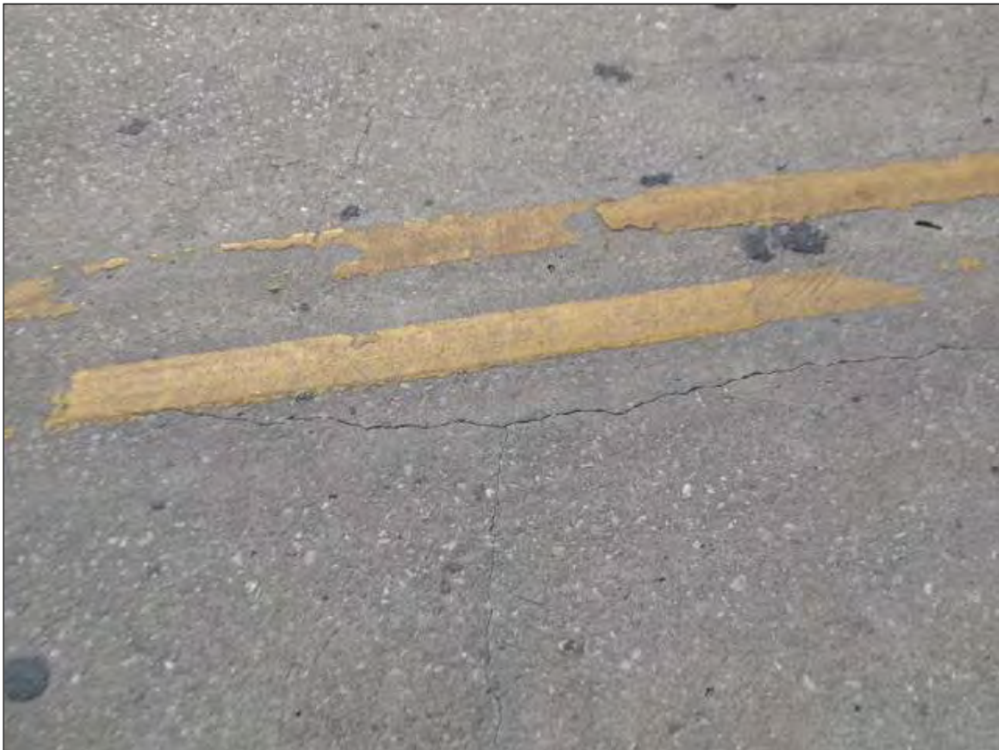
TRANSVERSE CRACKING/LONGITUDINAL CRACKING IN DECK IN ALL SPANS UP TO .040" WIDE
