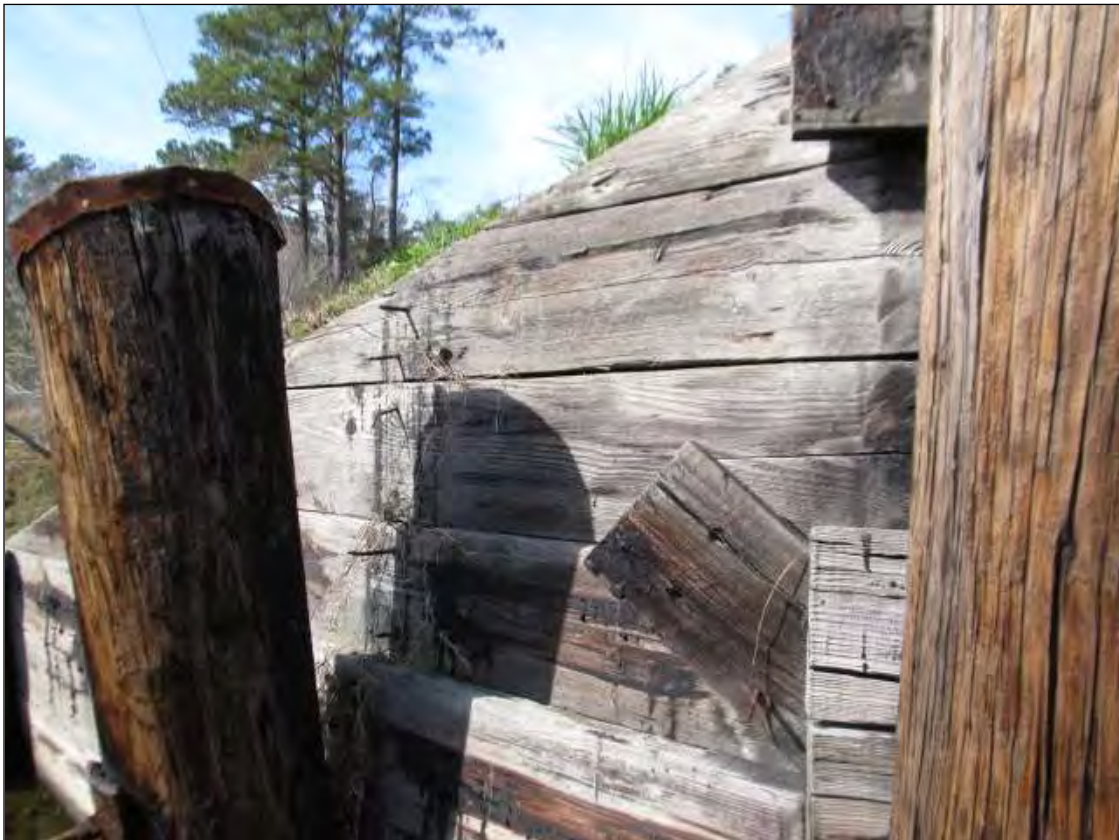
SOUTHWEST WINGWALL TOP 3 BOARDS ROLLED BACK AND DISPLACED UP TO 1"
