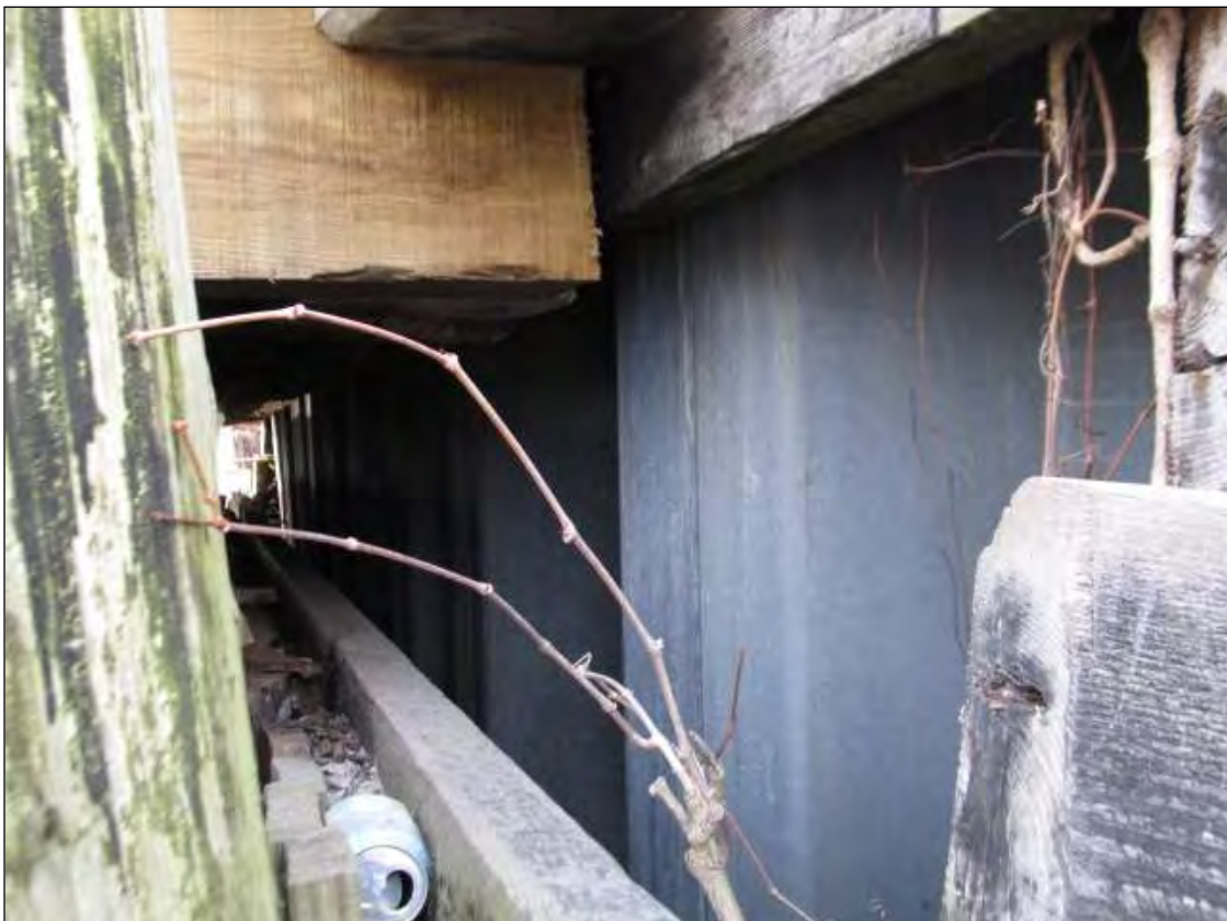
STEEL SHEET PILE IN PLACE BEHIND ORIGINAL BULKHEAD BOARDS AT END BENT 1.
