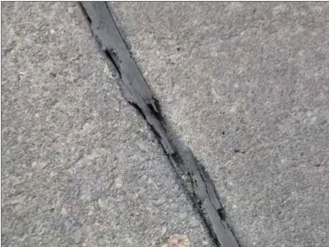
TOP SEAL ALONG JOINTS DETERIORATED
