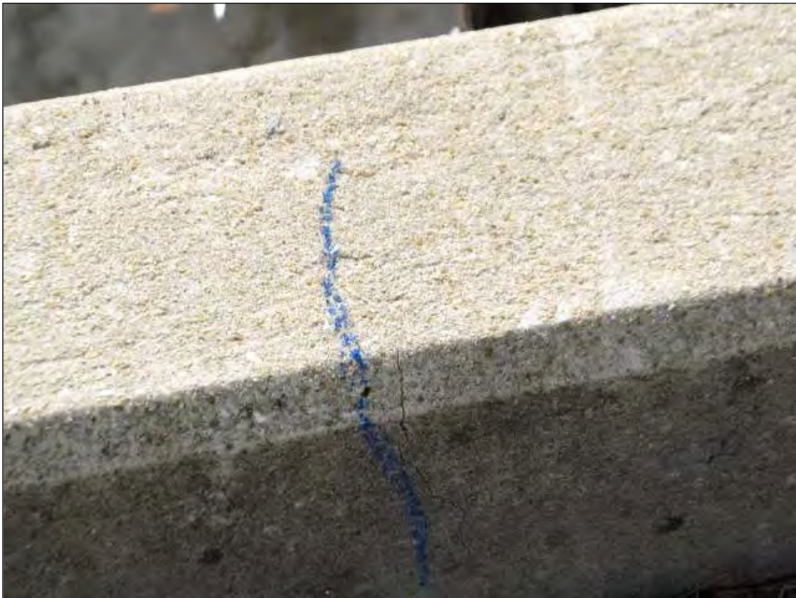
TRANSVERSE CRACKING/VERTICAL CRACKING ALONG CURBS
