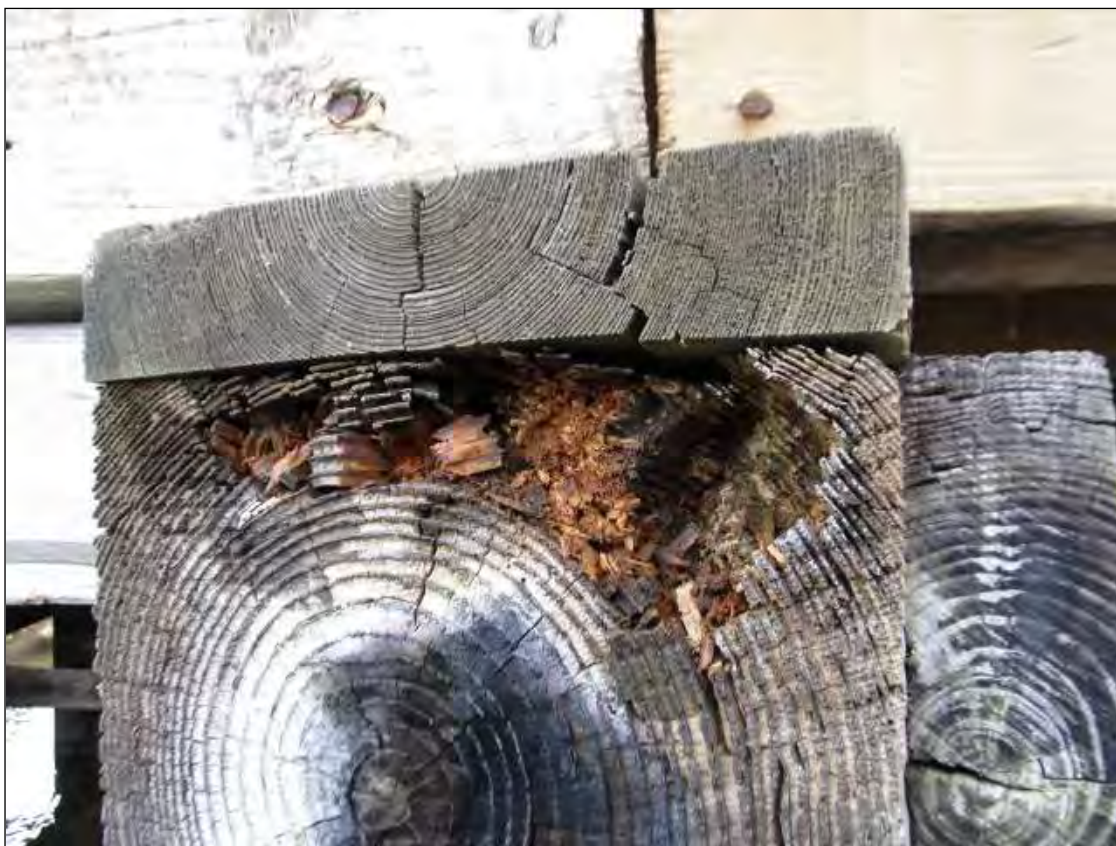
BENT 1 CAP AT NORTH END DECAYED AREA 10" WIDE X 2" TO 5" HIGH X 5" LONG.
