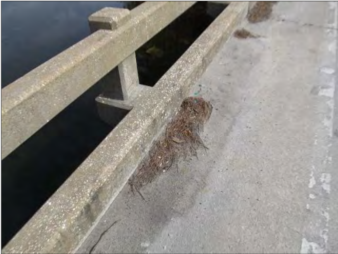
DEBRIS ALONG NORTH CURB BLOCKING DRAINS
