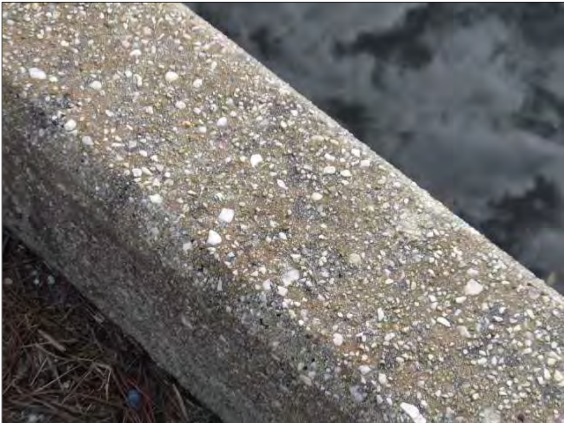
CURBS WEATHERED WITH EXPOSED AGGREGATE
