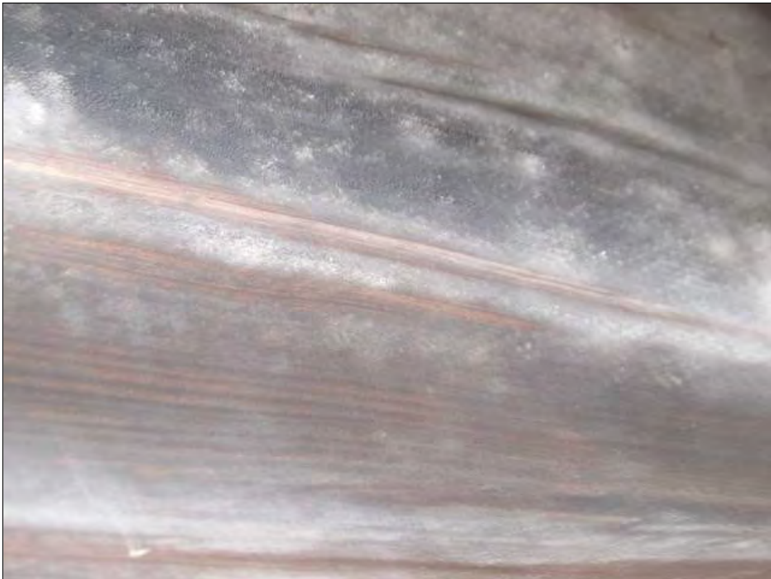
LONGITUDINAL CRACKING ALONG JOIST UP TO 1/8" WIDE
