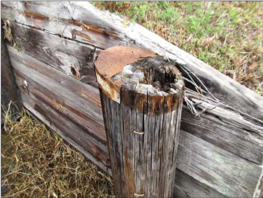
SOUTHEAST WINGPILE HOLLOW
