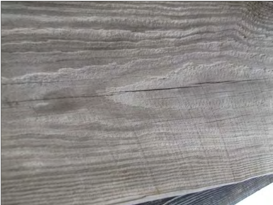
LONGITUDINAL CRACKING ALONG TIMBER CAPS UP TO 1/8" WIDE.
