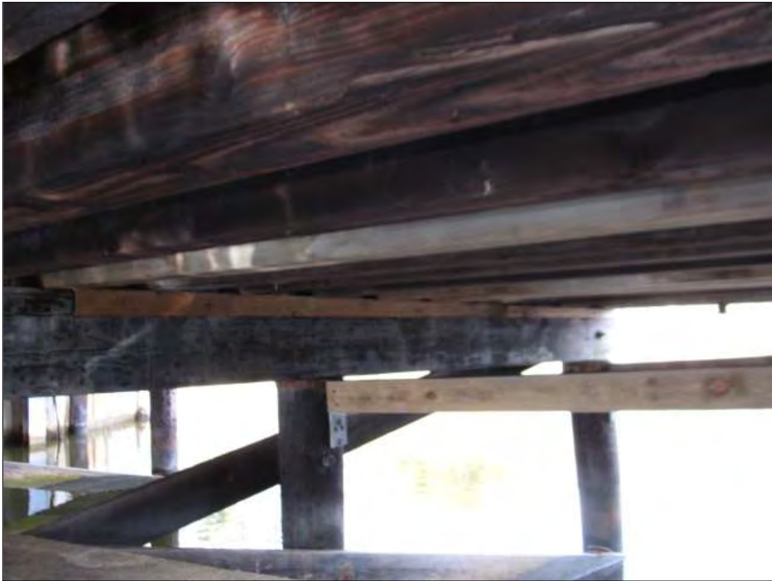
BENT 2 CROWN STRIP REPLACED WITH CCA MATERIAL AT JOIST 1-10
